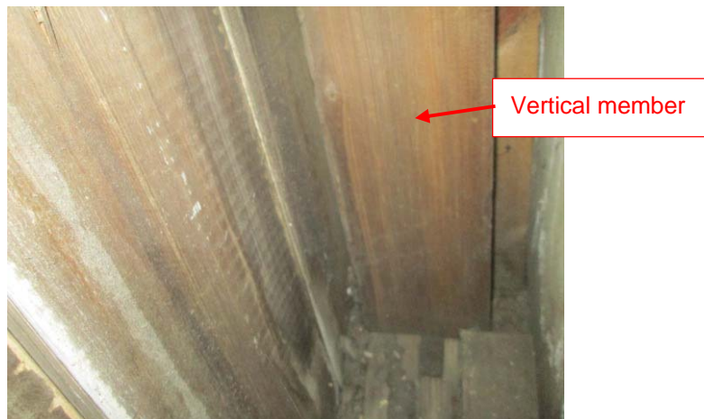
Figure 13: View in Panel 13 & 14 (staircase)
