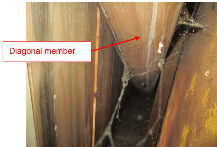
Figure 6: View towards Platform 1 in Panel 4
