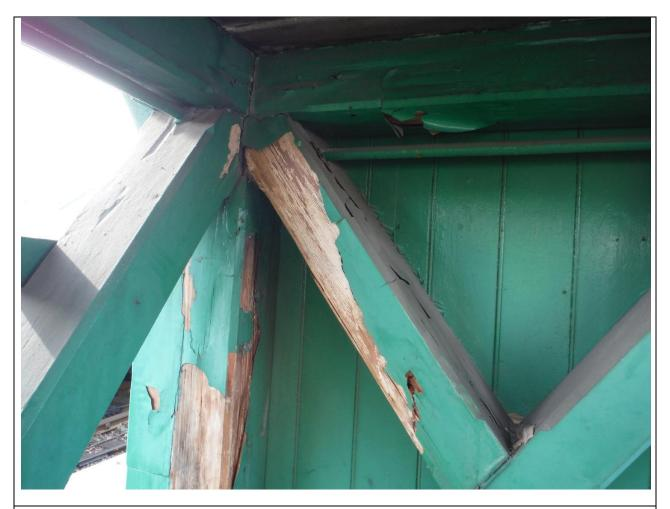
Photo 2: Dry rot to underside of 4 post support column diagonal brace (Platform 1)
