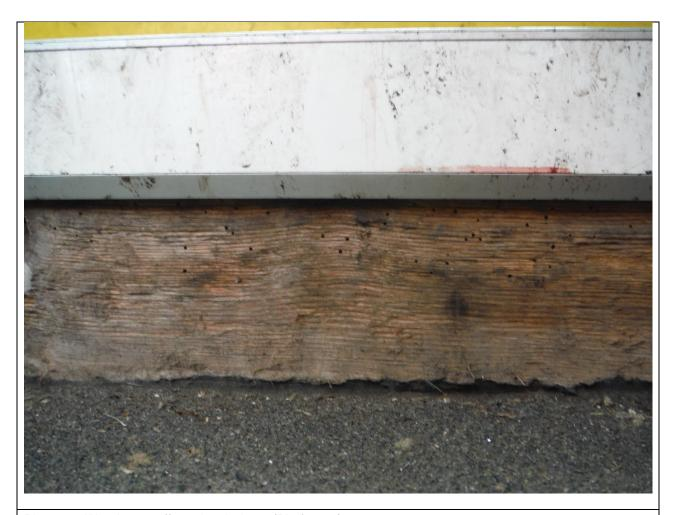
Photo 13: Woodworm affected stair risers (Platform 1)
