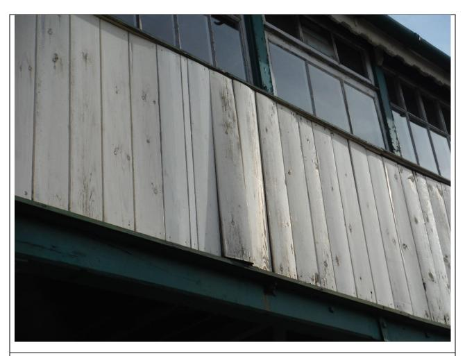
Photo 11: Swelling of timber cladding caused by rainfall. Cladding requires refixing to ensure it does not become dislodged in high winds (Platform 1)
