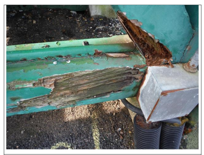
Photo 1: Wet rot to lower connection of 4 post support column diagonal brace (Platform 1)
