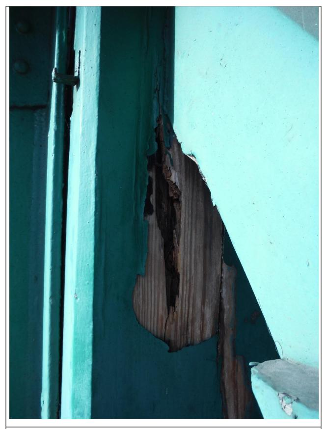
Photo 3: Dry rot to vertical face of 4 post support column diagonal brace (Platform 1)
