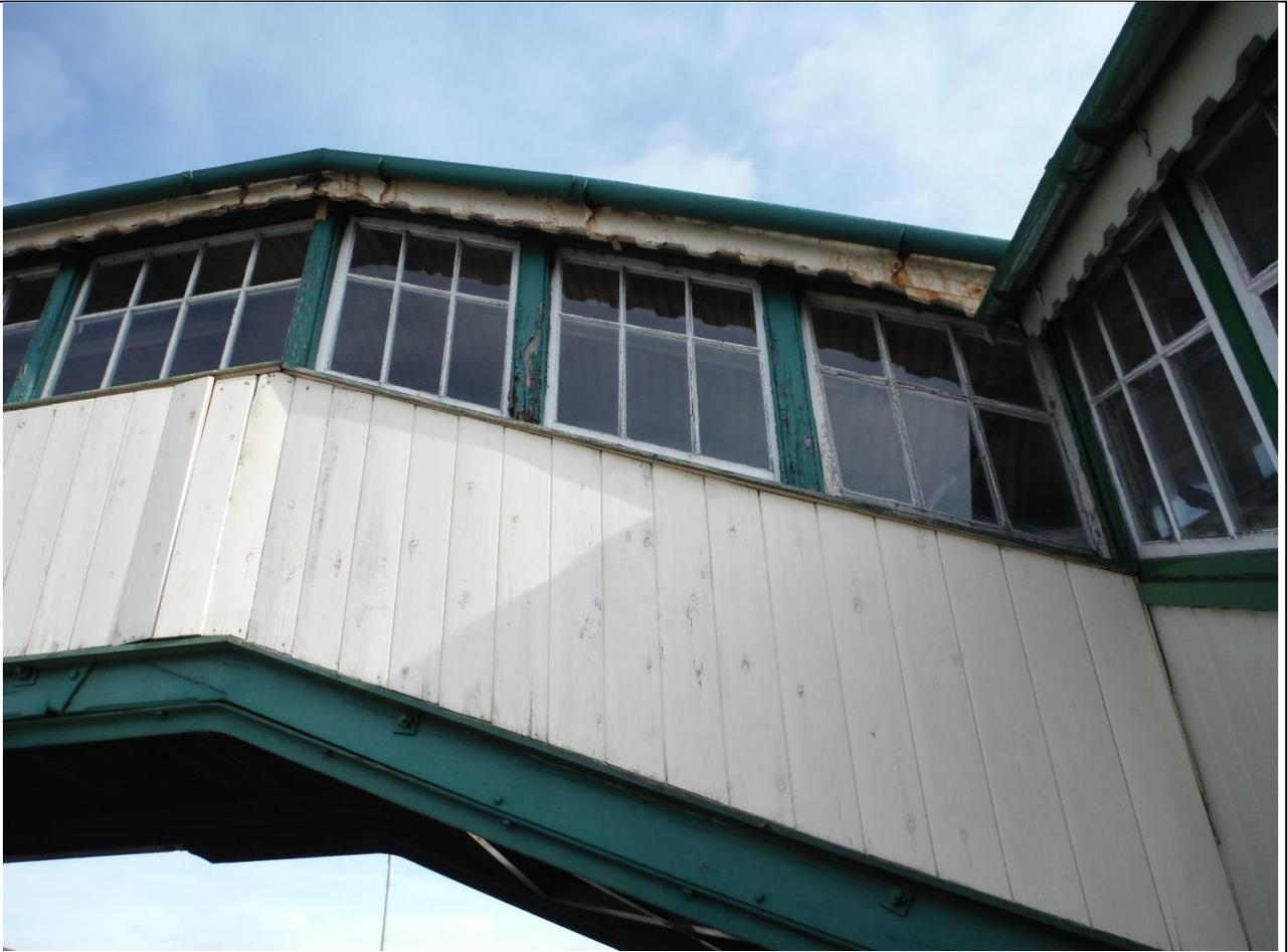
Photo 10: leaking gutter allowing water to spill onto country end face of the footbridge causing paint to peel and degrade timbers (Platform 2)
