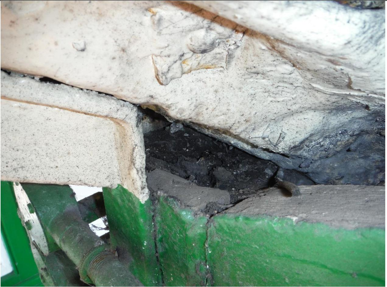
Photo 7: Wet rot to top of vertical roof support timber directly below leak (Platform 2)
