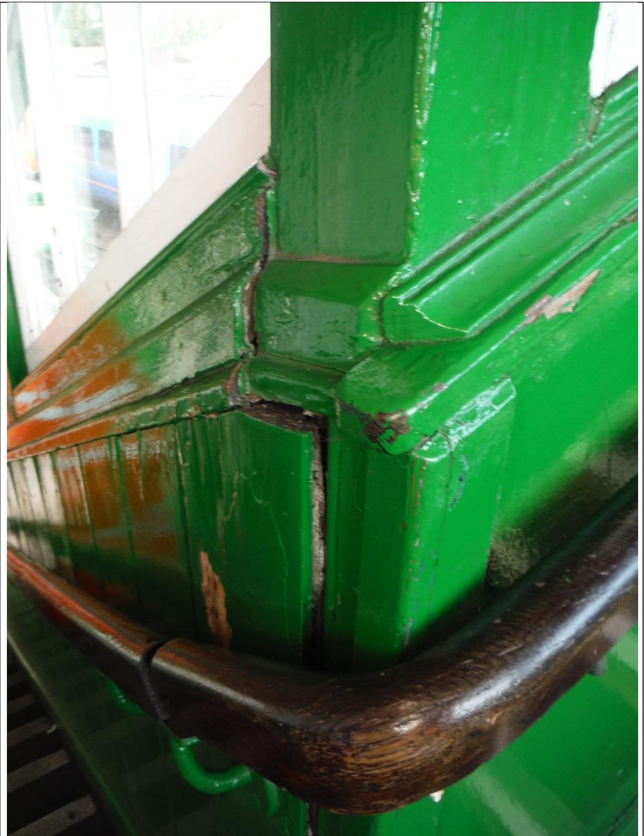
Photo 6: Roof leak above causing swelling and separation of stair corner joint (Platform 2)
