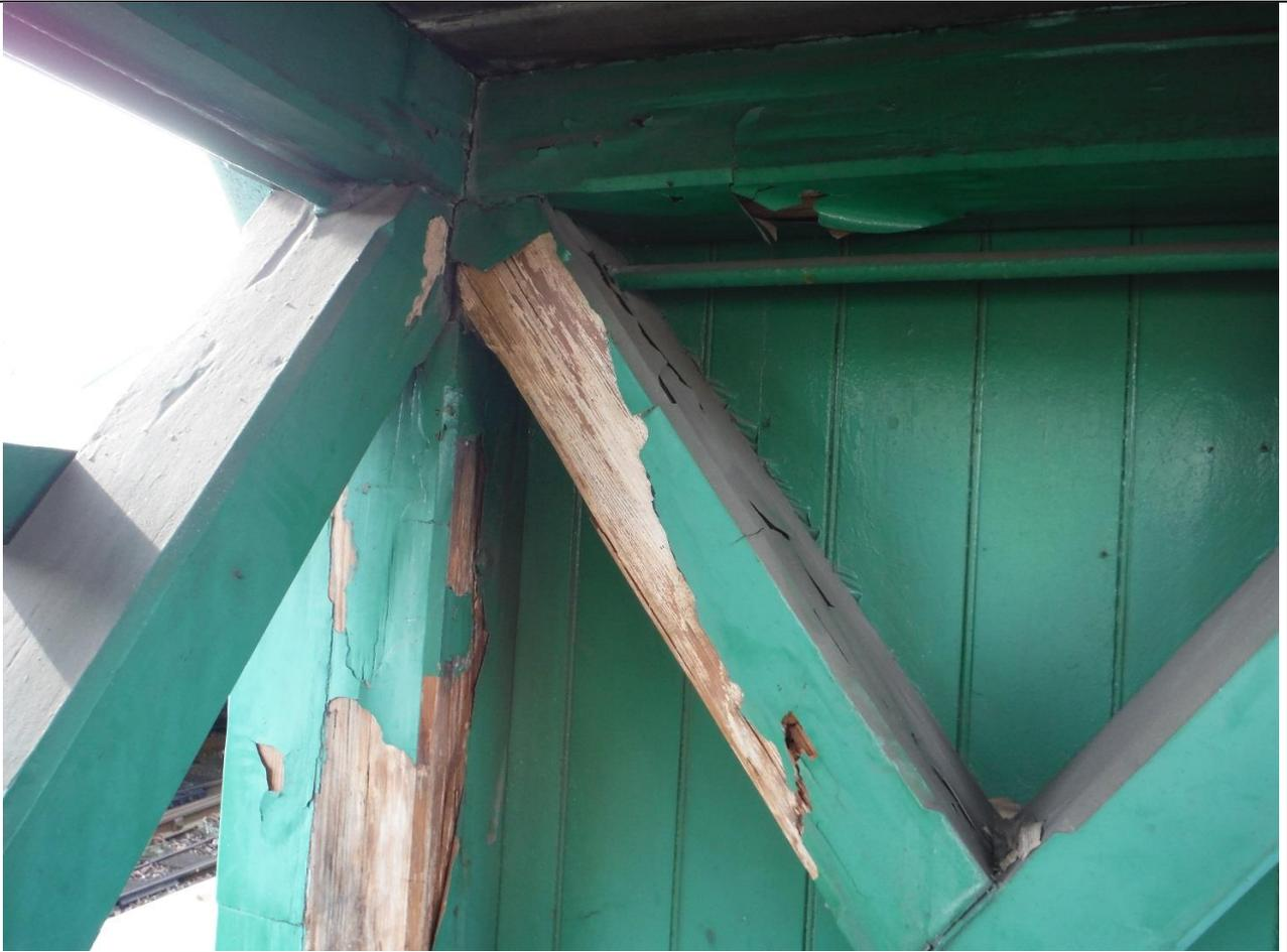
Photo 2: Dry rot to underside of 4 post support column diagonal brace (Platform 1)
