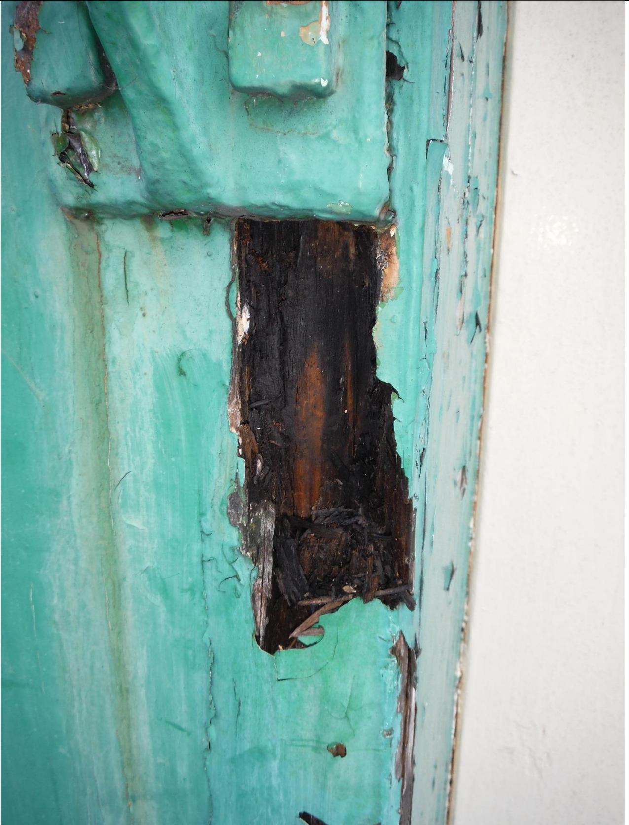
Photo 8: Wet rot of timber at steel T-section connection at westernmost corner directly below roof leak (Platform 2)
