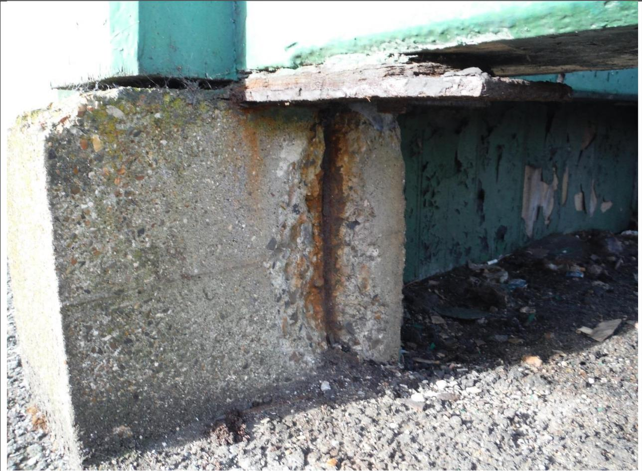
Photo 4: Minor spalling and corrosion of reinforcement at southernmost of 4 post column concrete base support (Platform 1)
